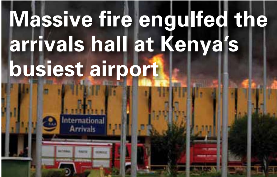
A fire at the Kenya's international airport gutted the international arrivals hall
